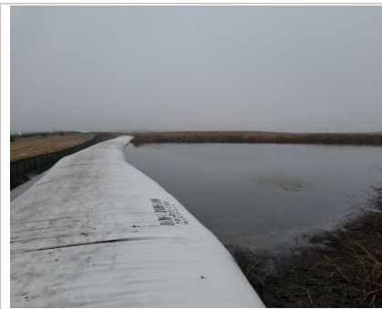
Description & Location KP-848+400
