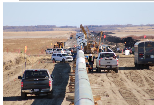
Description & Location: SSKP 877+500 Pipe Gang and Poor Boy Equipment needed to be cleaned Pipegang working through wetlands Photo facing east
