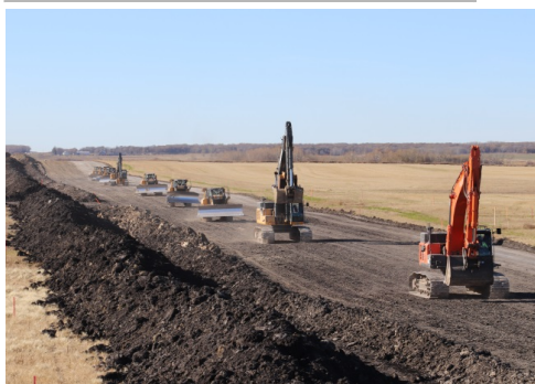
Description & Location: SSKP 890+800 Grade Crew Moving equipment ahead to next objective Getting lots of production done Photo facing northwest
