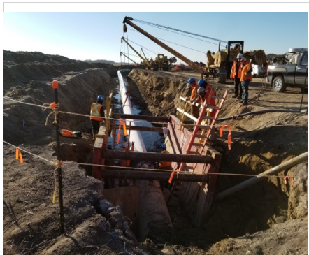
Dozers back filling behind the side Description & Location KP-822+125.6 booms.
