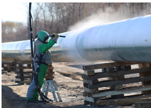
Description & Location: SSKP 853+900 Coating Mainline Sandblasting weld Preparing it for coating applicators Facing southeast
