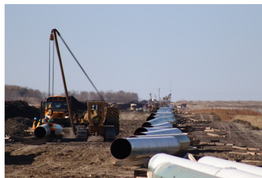
Description & Location: SSKP 879+750 Set-up crew to the left End Prep and Pipegang in background Pipe getting ready to be welded Facing west
